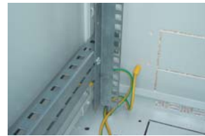
Bottom part of the rack—detail
